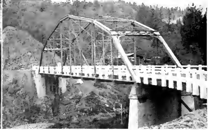
At left, old Salmon River Bridge at Somesbar, Siskiyou County. At right, how it looks rebuilt with steel salvaged from Eel River bridge at Scotia.
